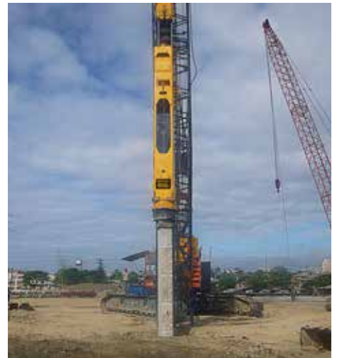
Above: CXL hydraulic piling hammers are designed for driving sheet piles, tube and H-piles, concrete piles, combi-wall and wooden piles.
