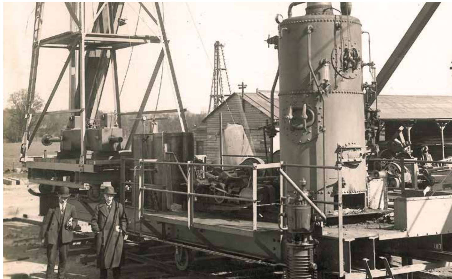
Below: An early BSP steam piling rig, Great Blakenham, 1920s.
