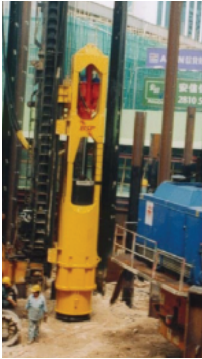
CG300 mounted on a piling rig
