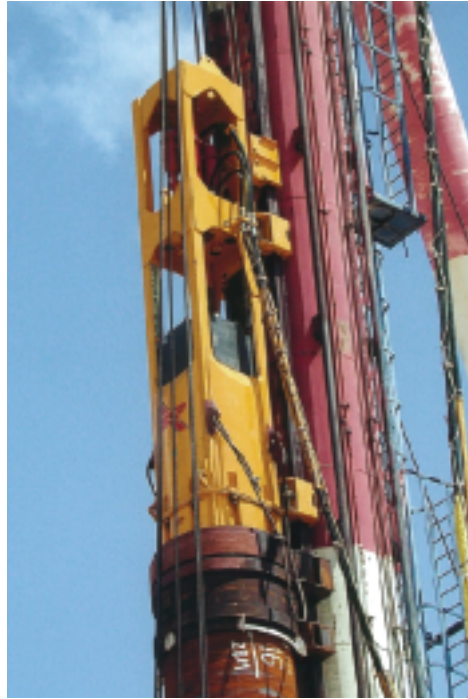
CG300, Leader mounted on a barge, driving steel tube piles
