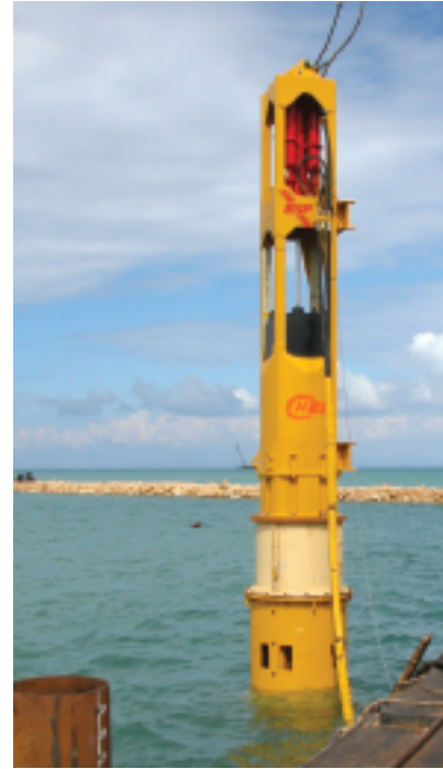
CG300, Crane suspended, driving steel tube bearing piles
