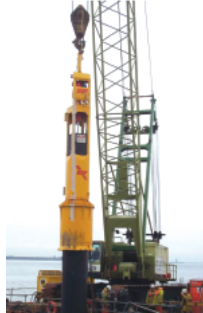
CX110, Crane suspended and fitted with tube guide
