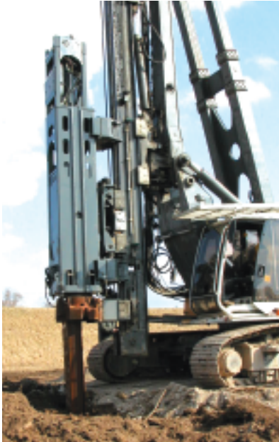
CX85, mounted on piling rig
