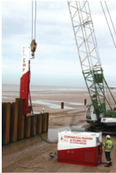
Above: Various SL30 Hammers fitted with legs and inserts for diving sheet piles. All are shown in crane suspended operation and powered by BSP Power Packs.
