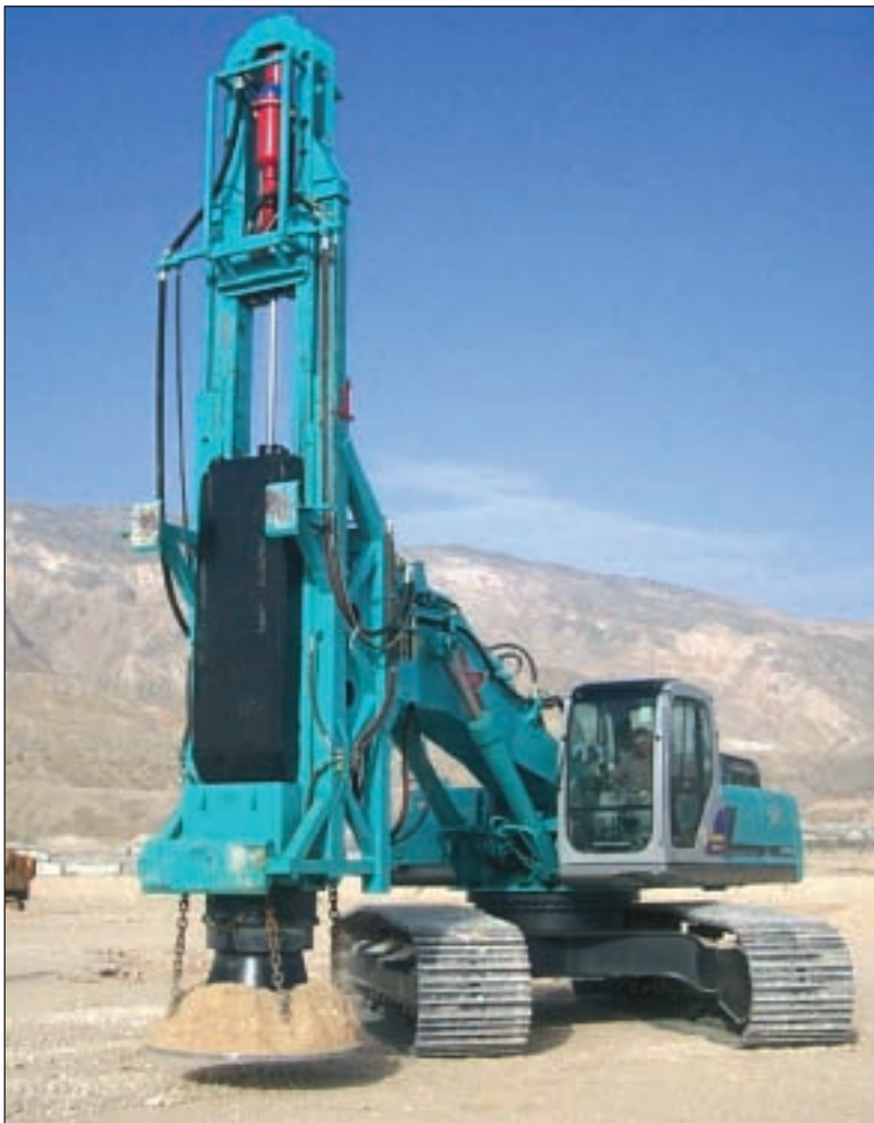
RIC 9000 mounted on Kobelco SK480
