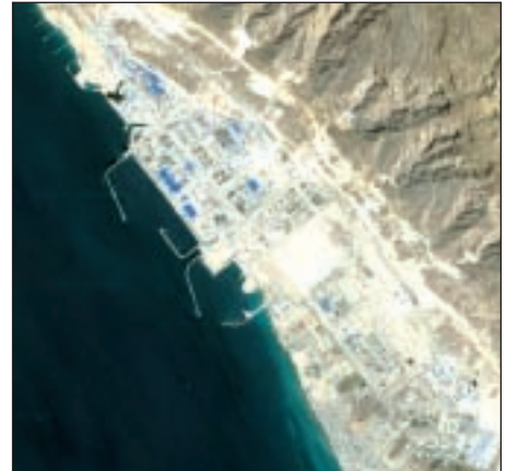
Arial view of land reclamation
