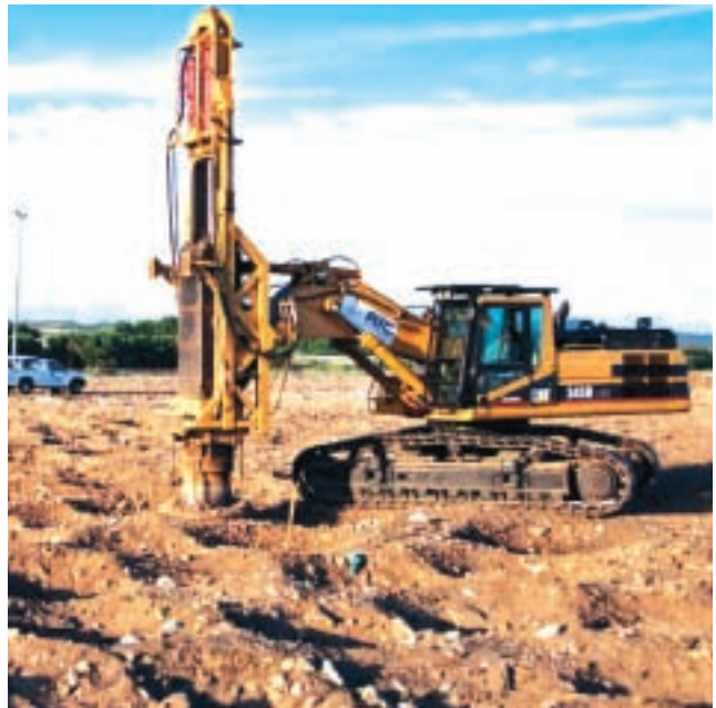
Compacting miscellaneous waste fill
