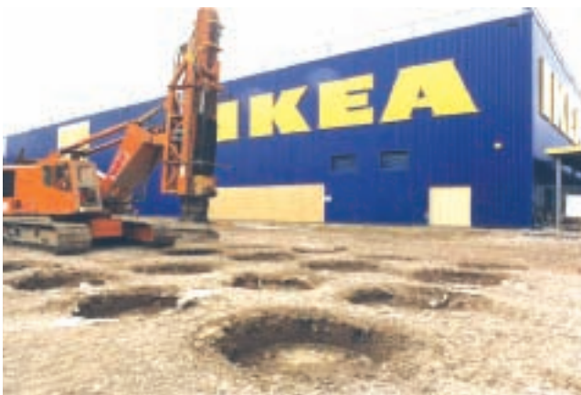
RIC 7000 in operation close to existing structure
