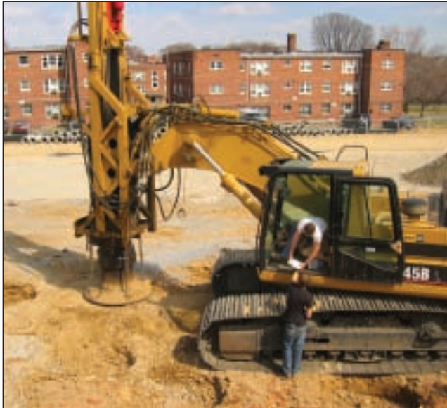
RIC improving the ground at site
