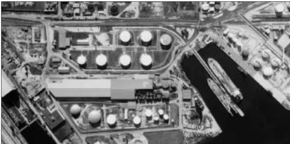
Arial view of Tampa Terminal Tank Farm
